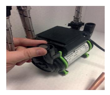
Once the pump and hoses are in place, it will be possible to mark or measure how much of the inlet pipework will need to be trimmed back using a pipeslice or cutter.
