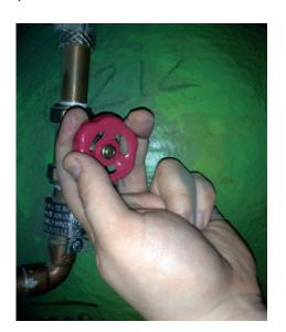
The existing push - fit hoses can now be removed by pushing the gripper ring towards the hose and sliding the body away from the pipe - depending on the installation the outlet hoses may be suitable for the new pump without changing them.
