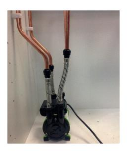
When everything is watertight, open any outlets so that a natural flow under gravity can fill the system, it can be plugged in, or the plug removed and wired into a fused spur so that the pump can be fully tested.
