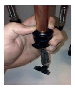
The new pump can now be unpacked, the noise reducing rubber feet fitted and the pump offered up to the installation - if the installation will allow, the outlet flat washer can be fitted and the pump connected to the outlet pipework. If the installation will not allow this, the new, longer hoses may be used following the next steps...
