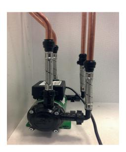
2 Usually the pump will have its own isolating valves to turn the water supply off to the pump.
